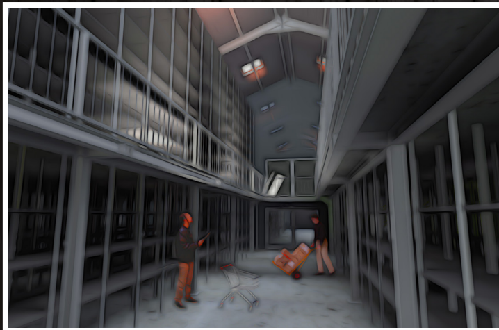
Work on the new warehouse will be completed next year
